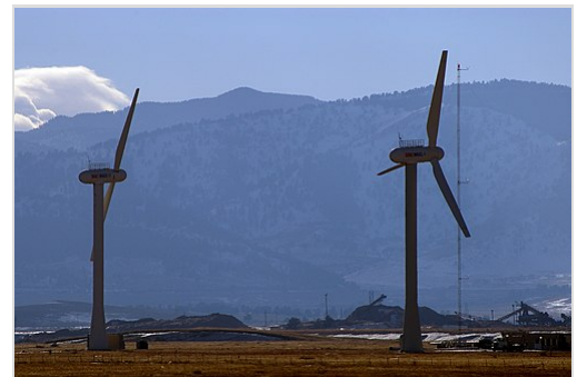
The main research wind turbines at NREL
